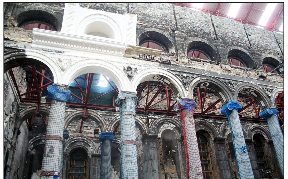
Picture shows trial plasterwork undertaken in summer of 2011.
